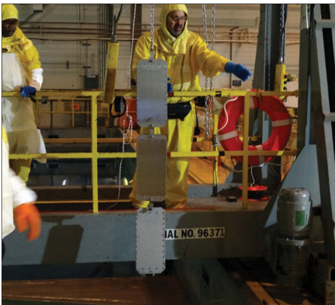
Fig. 6. Coupon tree removal (left) and rack module removal (right) from the Zion SFP.
