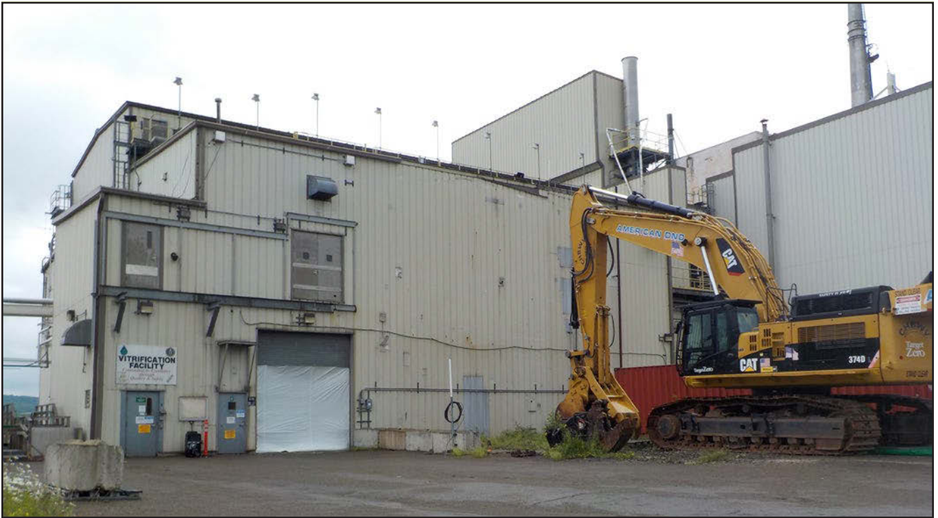
The vitrification plant before crews began demolition work.
