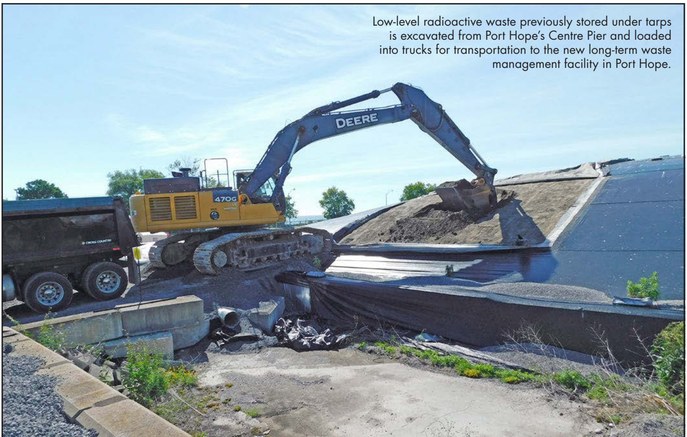
Construction of the baseliner cells of the Port Hope Project engineered waste storage facility began last year. The baseliner is a multilayered system used to isolate the waste from the environment. Materials such as clay, geosynthetic liner, and aggregate are sourced from regional suppliers.
